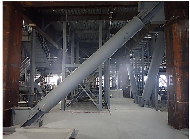
Fig. 11 Cruciform plasticizing section FMS alloy brace dampers mounted at the Chunichi Building.
