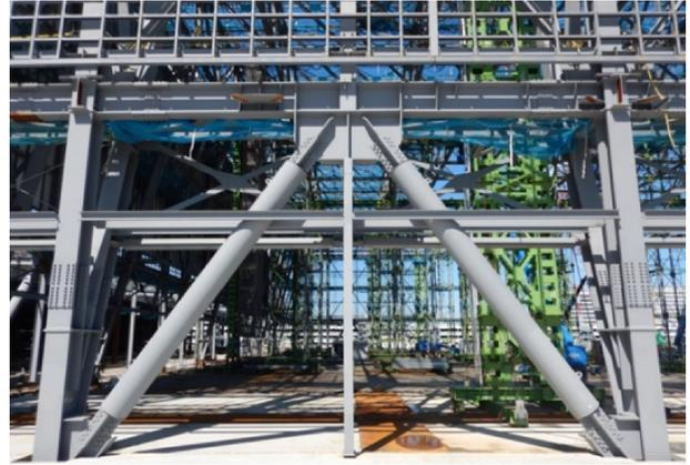
Fig. 10 Flat plasticizing section FMS alloy brace dampers mounted at the Aichi International Exhibition Center.
